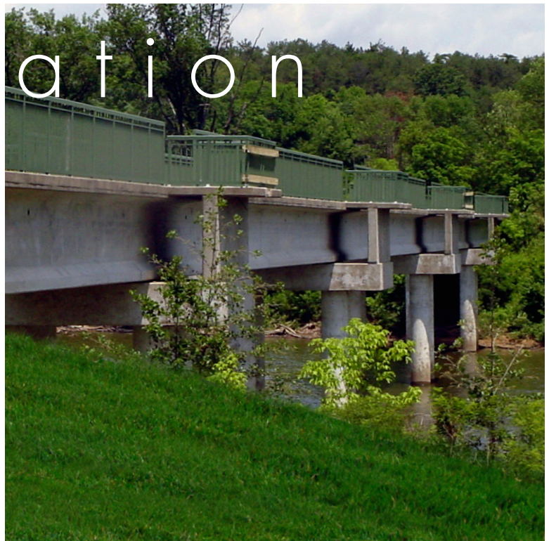
Winton Woods East Bridge, Cincinnati, OH
