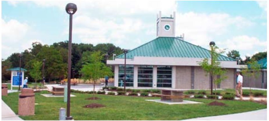
I-75 Rest Areas, Butler County
