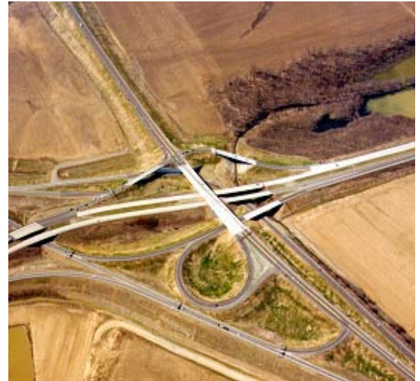
Our Transportation & Municipal Group provides expertise in both complex and non-complex roadway design.
