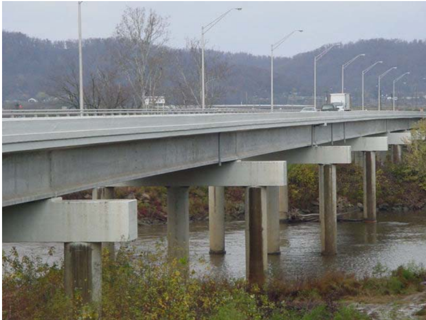
I-girder bridge beams
