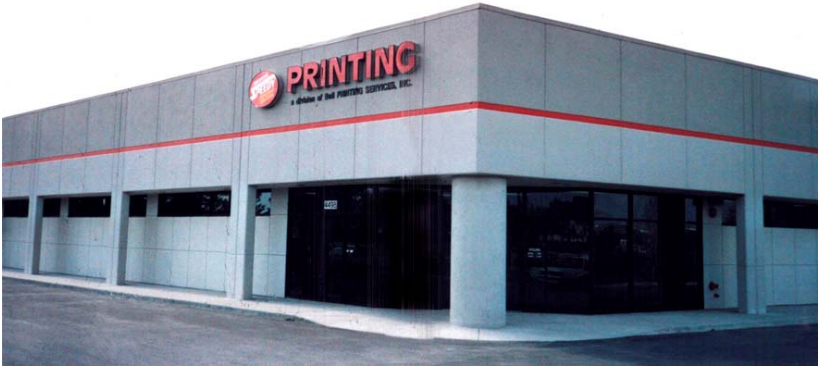
Precast tilt wall panel construction for buildings
